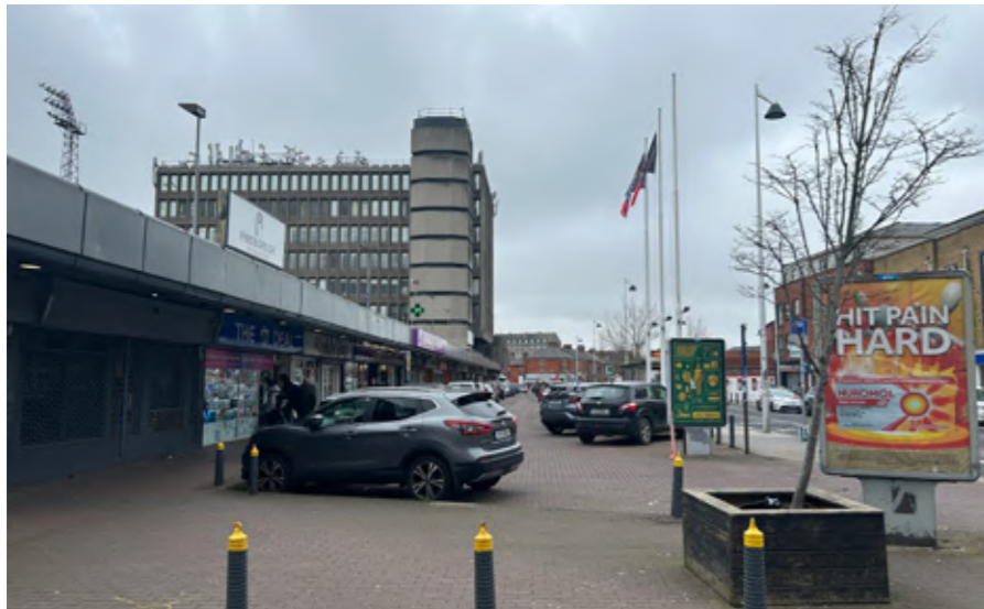
Fig. 4 View looking towards shop fronts along Phibsborough Road
