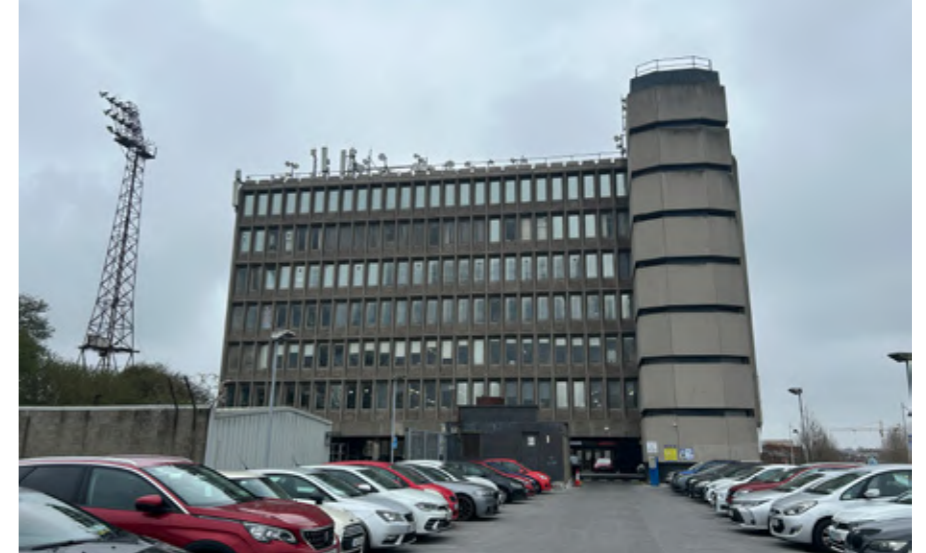
Fig. 3 View from roof level car park
