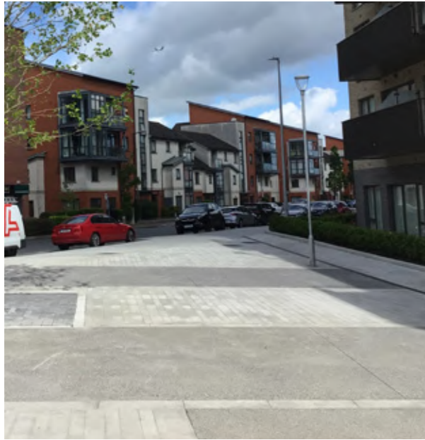
Exposed Aggregate Panels with natural stone banding
