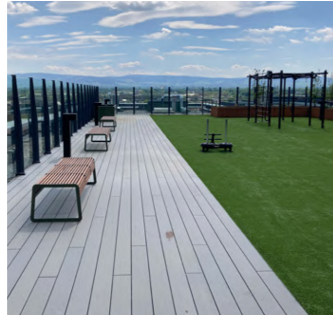
Roof terrace: Composite decking & artificial lawn
