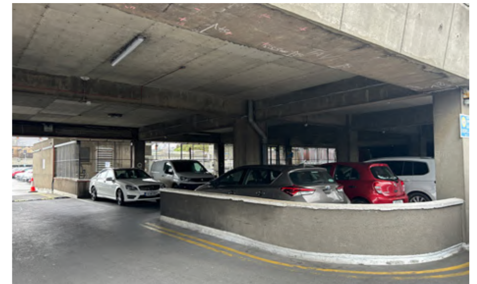
Fig.12 View from roof level car park
