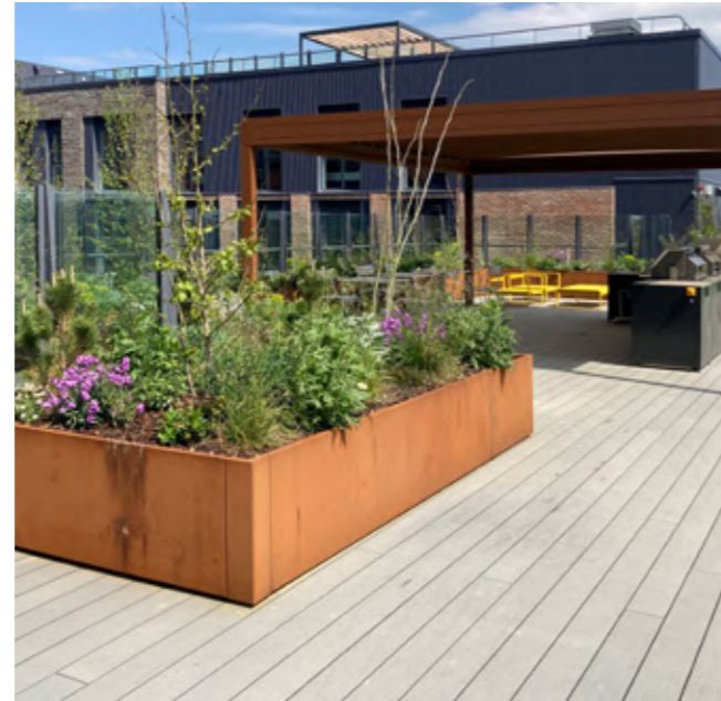
Roof terrace: Steel Edge raised planters
