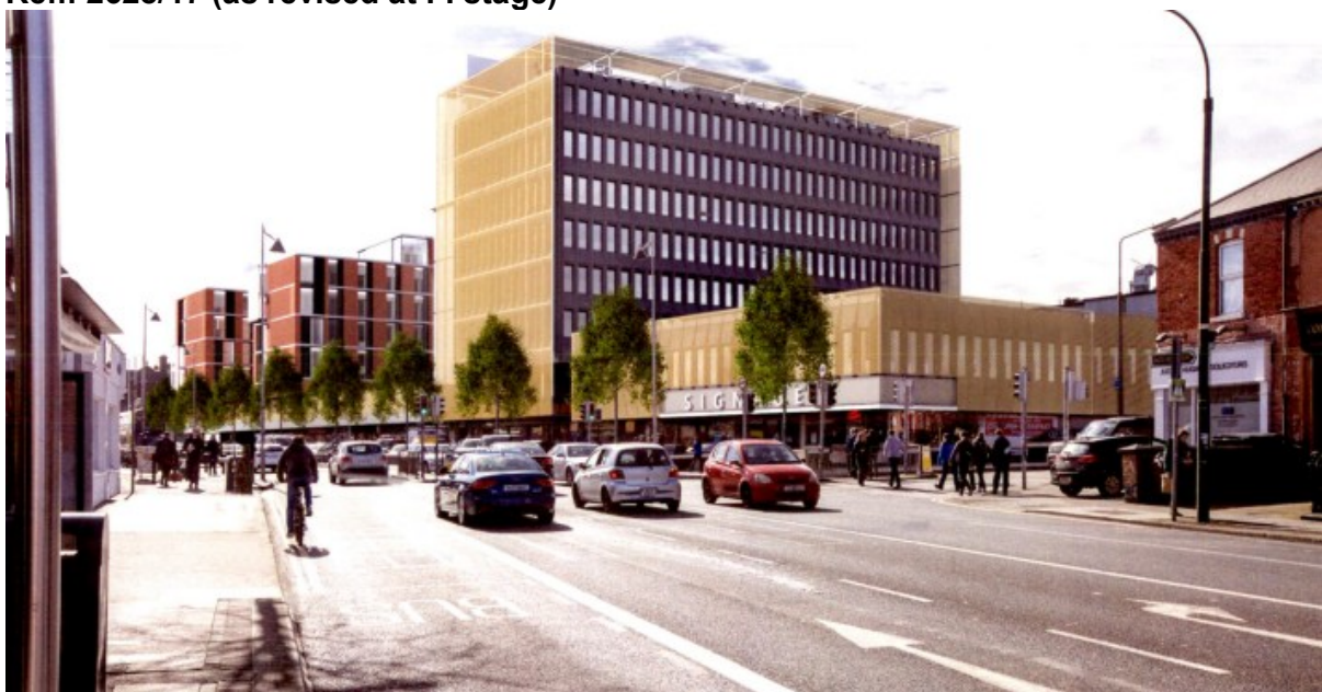
Figure 3.1: Proposed View of Development under ABP Ref.: 300241-17 / DCC Reg. Ref.: 2628/17 (as revised at FI stage)
