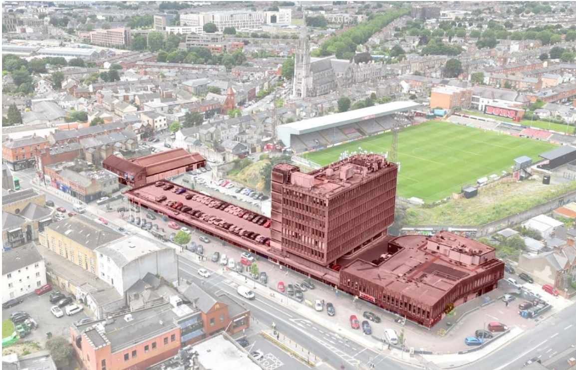
Figure 2.3: Bird’s-Eye View of existing buildings on site
